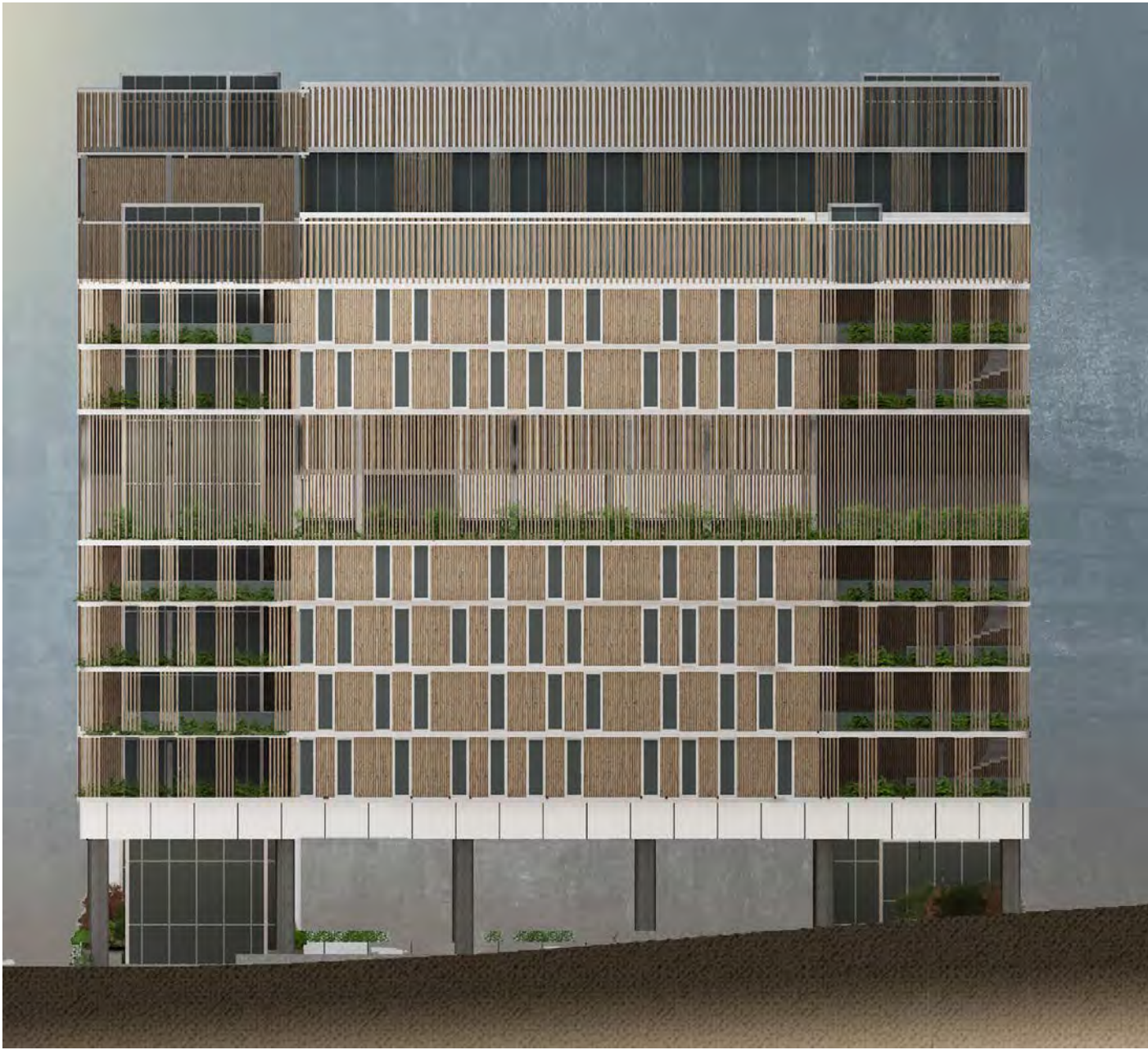
INTERIOR OF COURT YARD
